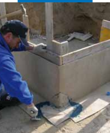
Grouting a gap in correspondence with a corner of the sheet with Mapeproof Mastic
