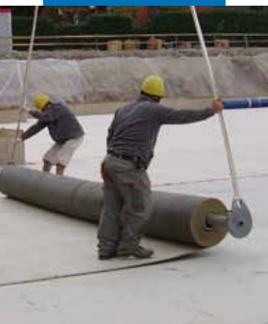
Waterproofing a horizontal surface with Mapeproof LW
