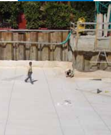
Waterproofing of structures below ground level against sheet piles
