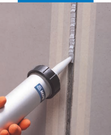
Application of Mapectex PU40
