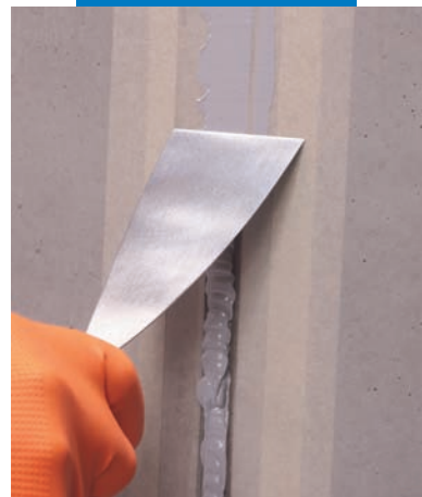
Smoothing over Mapecflex PU40
