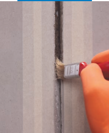
Application of Primer AS
