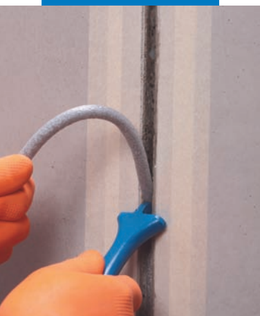
Inserting Mapefoam inside the joint
