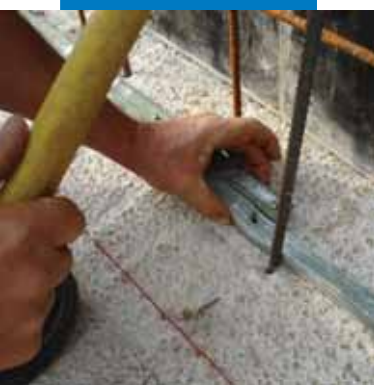
Fixing Idrostop B25 in place
